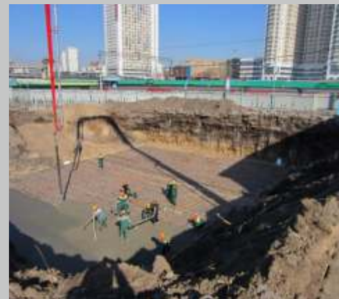
Moscow, Bryanskiy Post st., vl.7, Pit wall and retaining wall of piles and Atlant anchors
