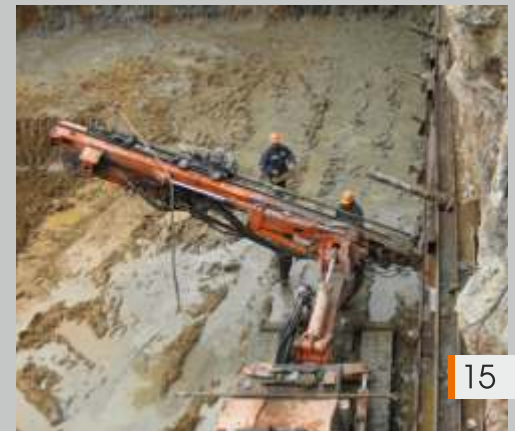
Reinforcement of pit wall Moscow region, Pushkino, Chekhova St.
