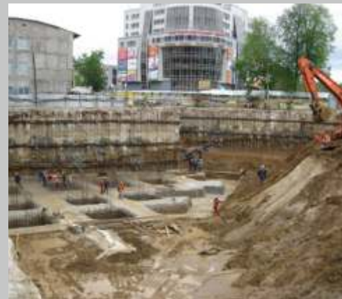
Reinforcement of pit wall Moscow region, Pushkino, Chekhova St.
