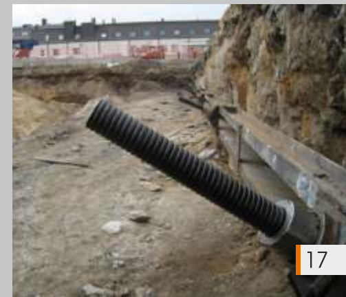
Moscow, Bryanskiy Post st., vl.7, Pit wall and retaining wall of piles and Atlant anchors
